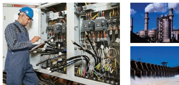
Supports high voltage systems around the world
