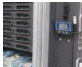
Recording temperature and humidity in a server room
